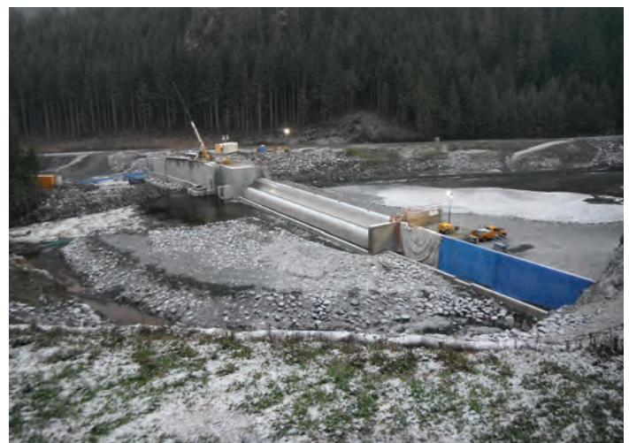
Kokish HEP, 45 MW, Port McNeil, B.C.
